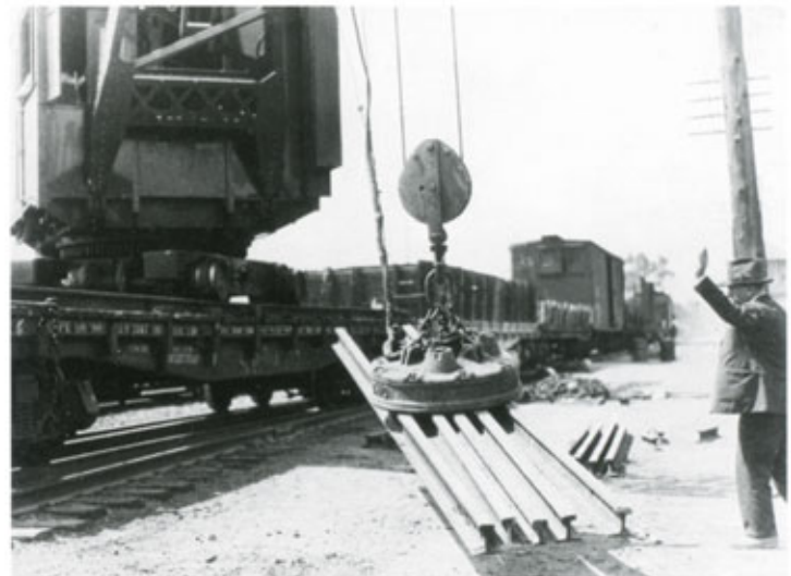
36" Ohio Magnetics magnet lifts railroad track Southern Pennsylvania Railroad - 1919
